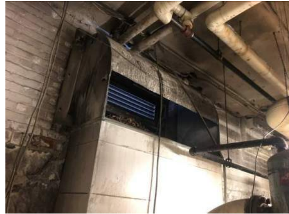
Existing Combustion Air Duct, Low Opening (left) and High Opening (right)
