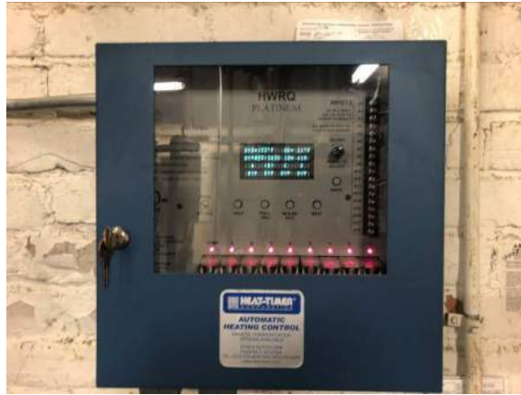
Boiler Controller
