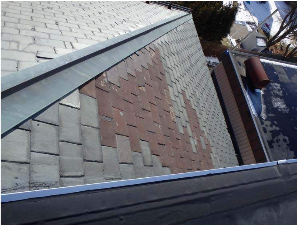
Figure 20. Area of replacement slate on southwestern slope
