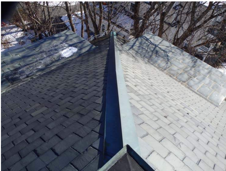
Figure 22. Red copper flat seamed dormer roofs
