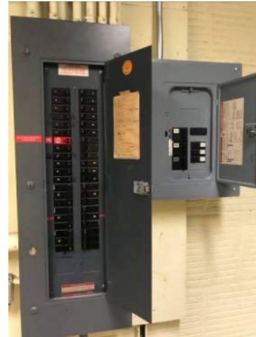
Normal/Emergency Panel/Subpanel
