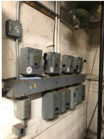
Starters & Disconnect Switches
