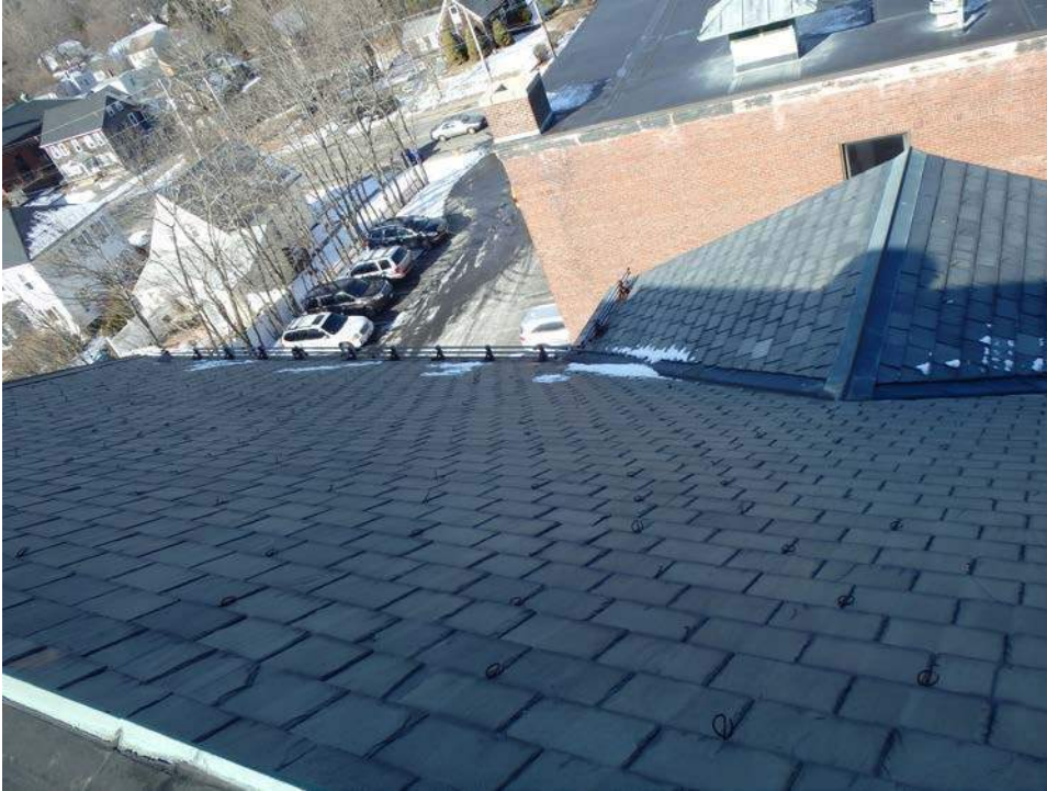
Figure 19. Slate roof showing typical intact condition
