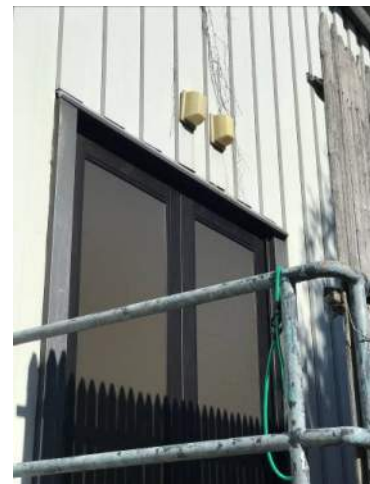
Wall Scones at Rear Parking Door
