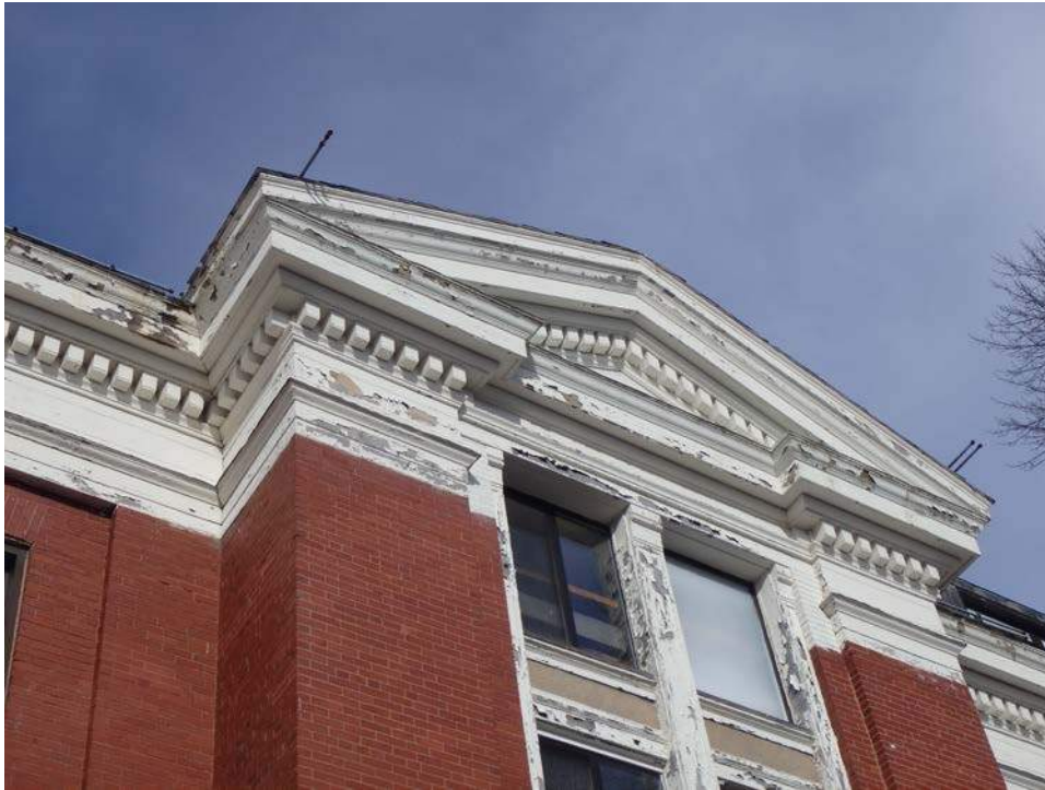
Figure 23. Snow rails loose from bracket and projecting beyond roof edge
