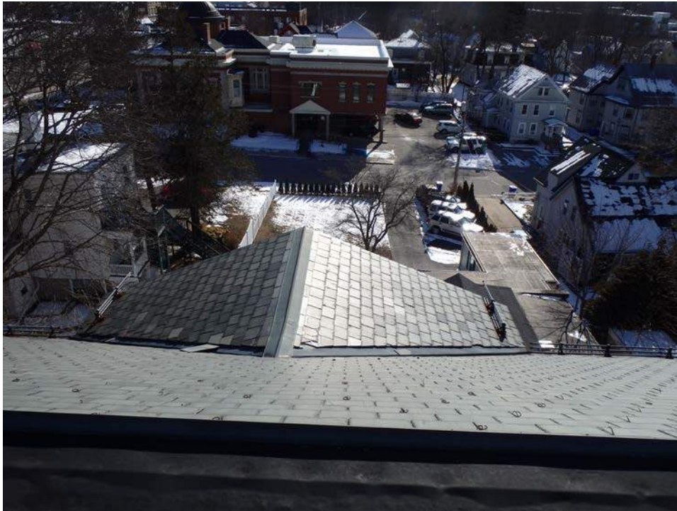
Figure 21. Red copper ridge and valley flashing; note snowrails at roof edge
