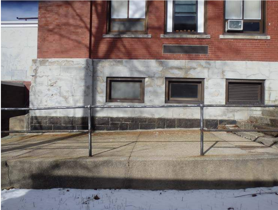
Figure 13. Area of exposed granite foundation stones
