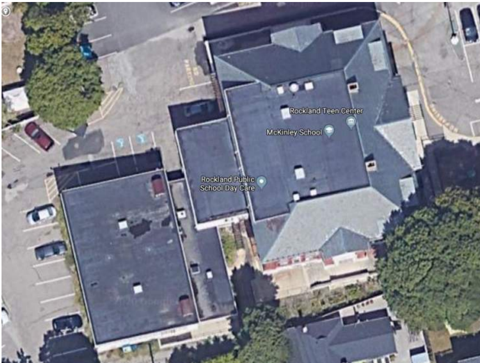
Figure 18. Google roof view showing sloped slate roofs and flat epdm roofs
