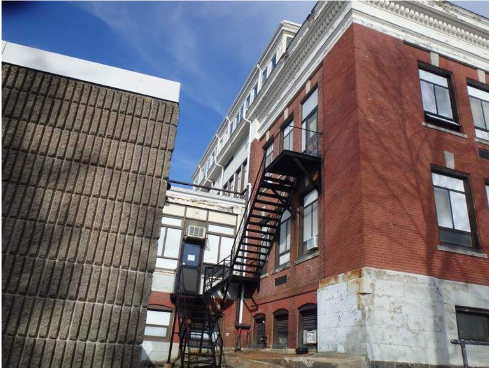
Figure 7. Fire escape and associated rust staining
