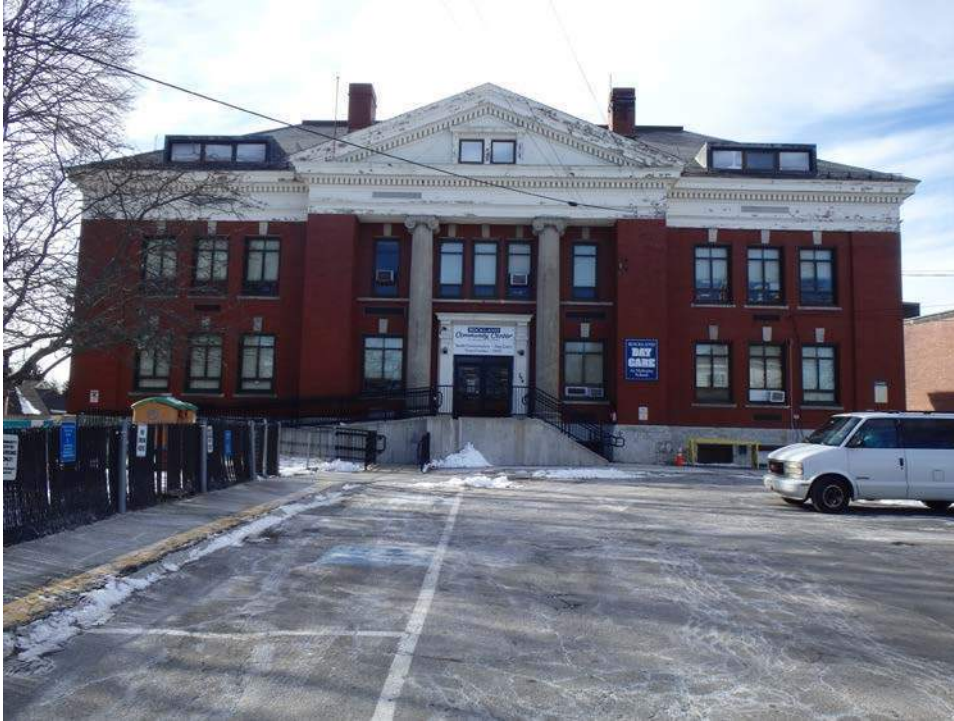
Figure 1. East elevation, front façade
