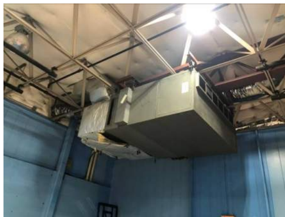
Gymnasium – Heating & Ventilation Units
