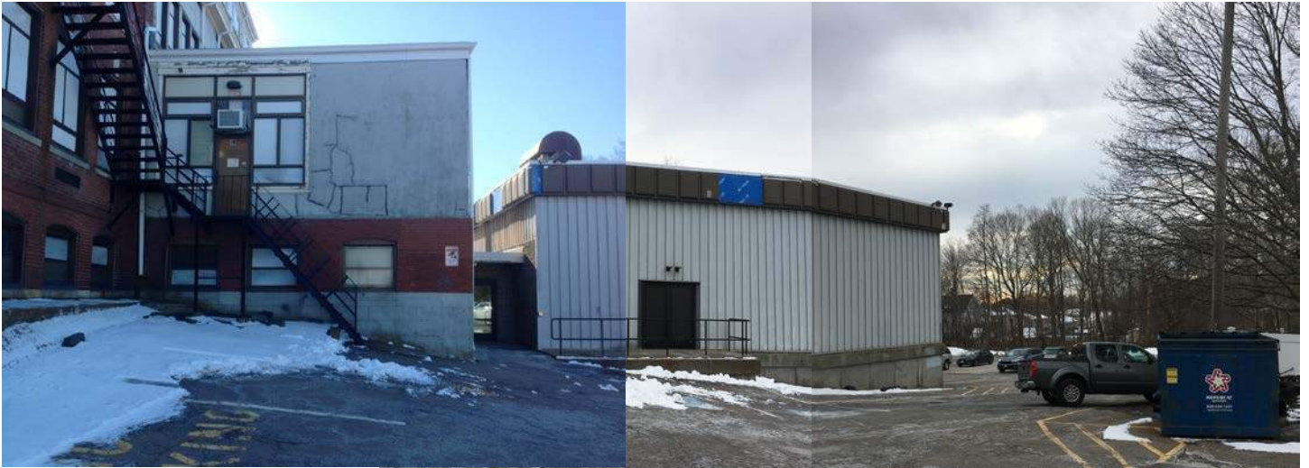
Driveway connecting front and rear parking lots
